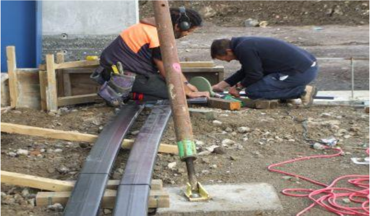
HDPE Poly lock fabrication.
