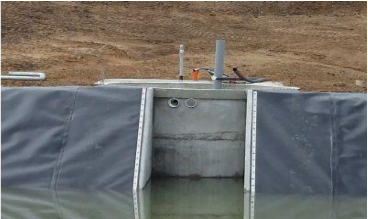
Stainless Steel – Concrete Attachment Detail.
