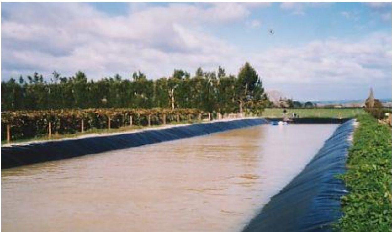
Completed Liner at Kiwifruit Orchard.
