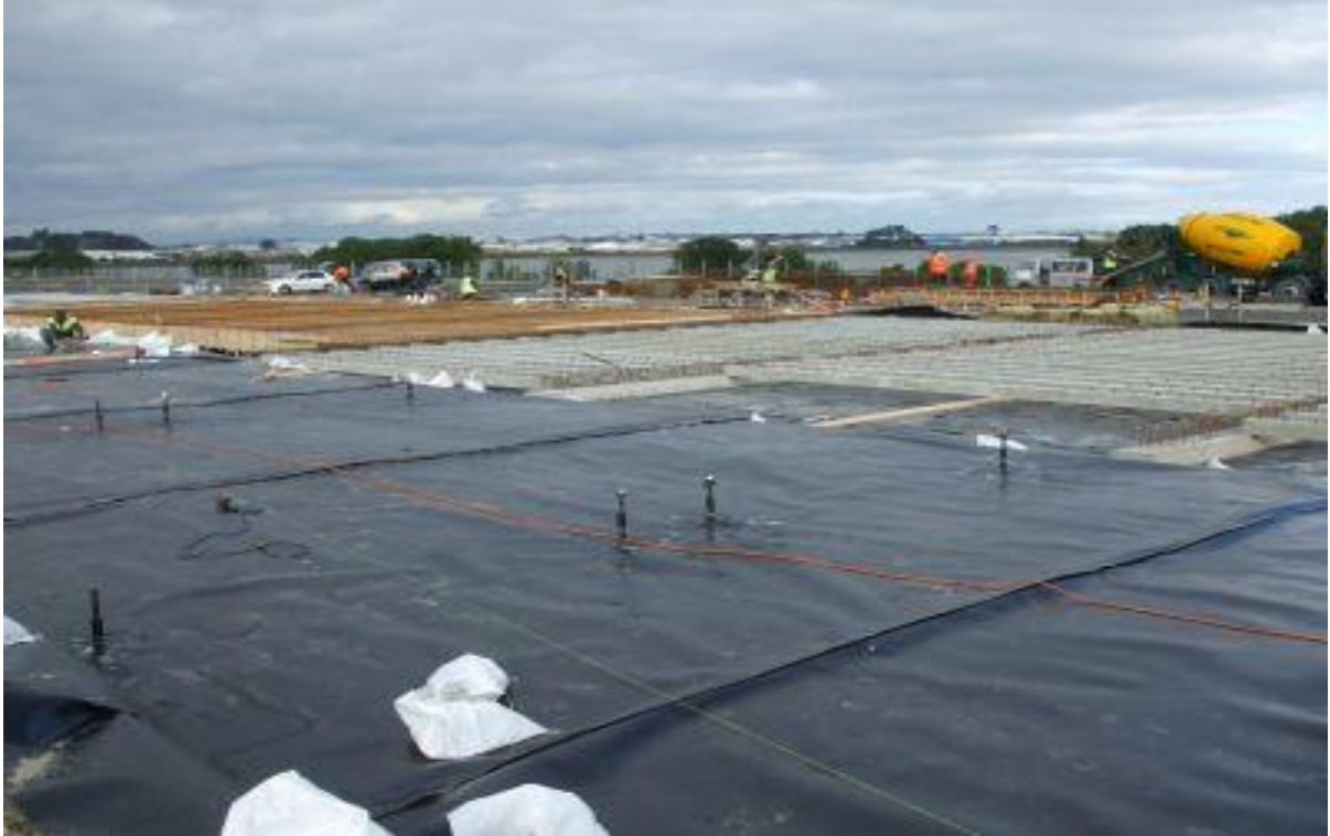
Installation of commercial gas barrier membrane
