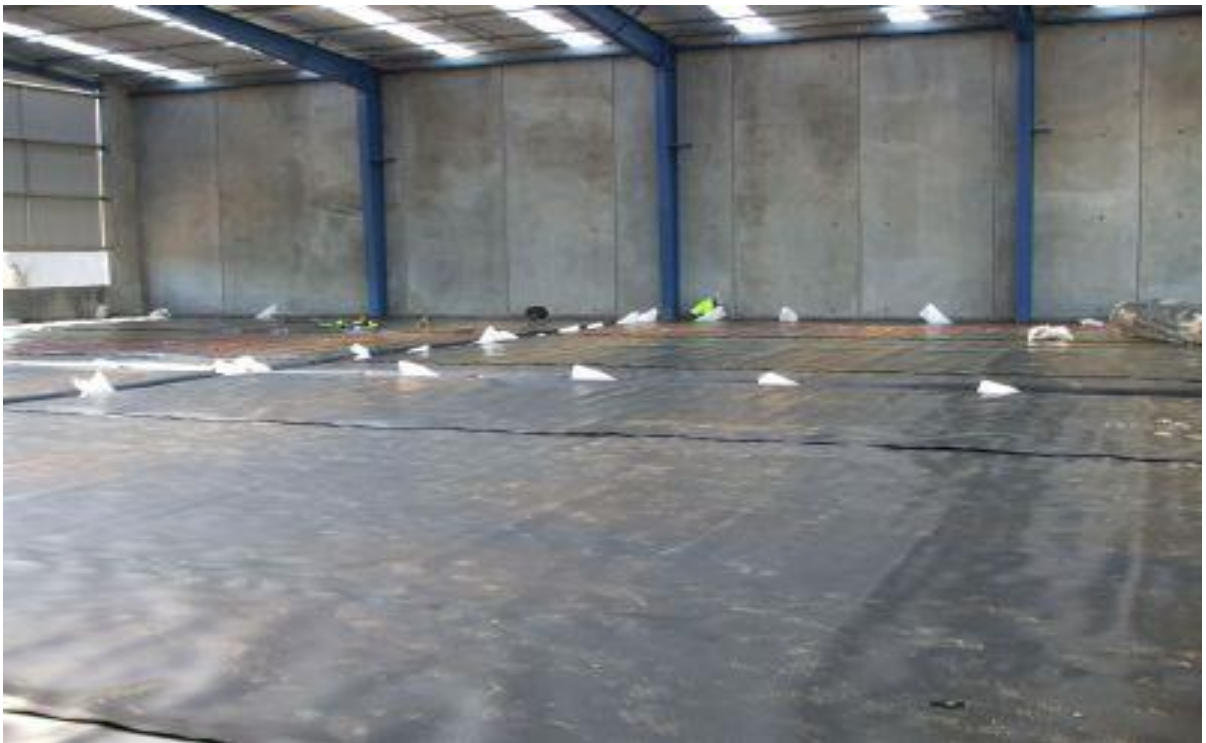
Installation of Industrial Warehouse Gas Barrier Membrane.
