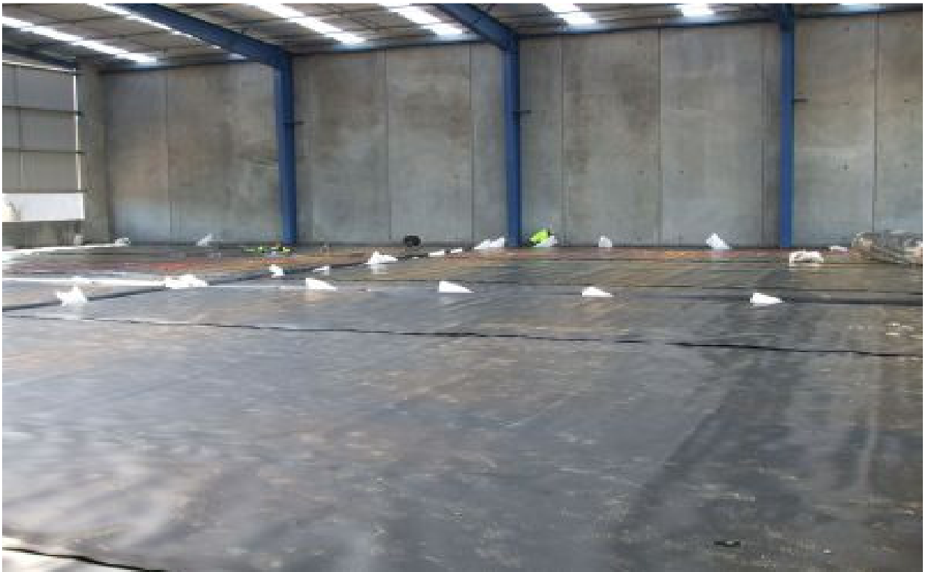
Installation of Industrial Warehouse Gas Barrier Membrane.
