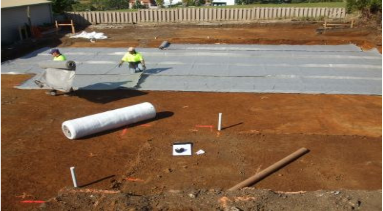
Installation of gas transmitting geonet.
