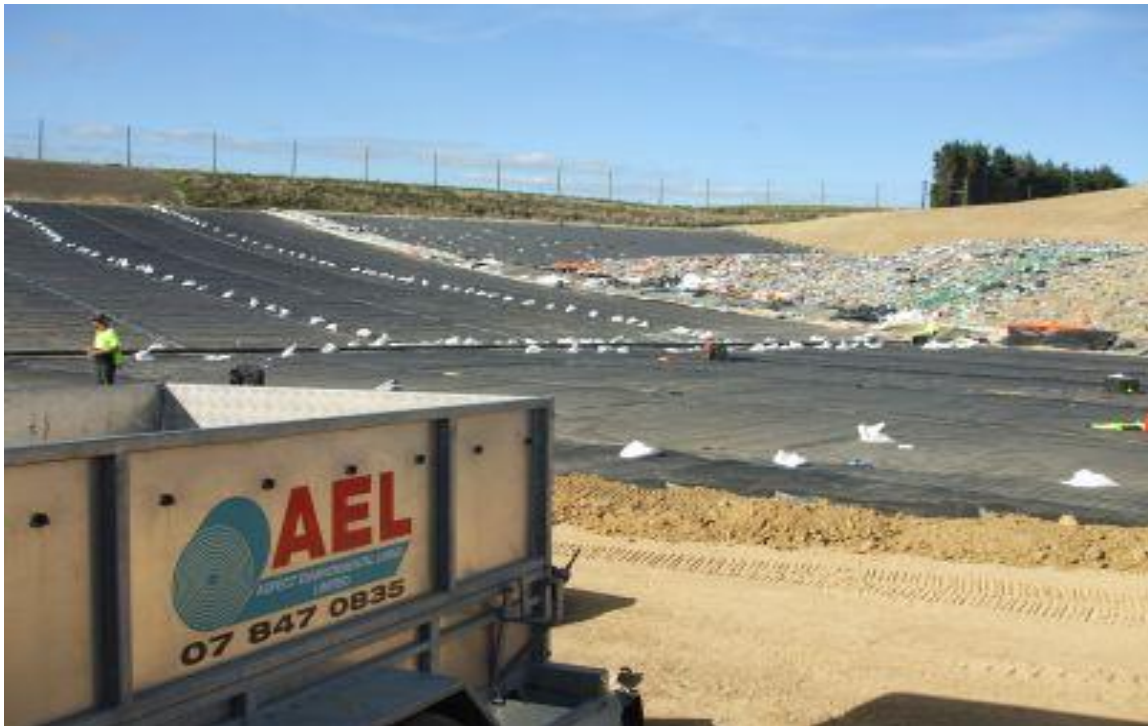
Landfill Cell – Liner Extension Project
