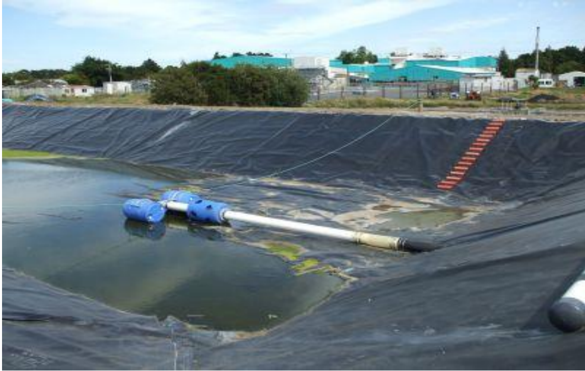
Waste Water Pond
