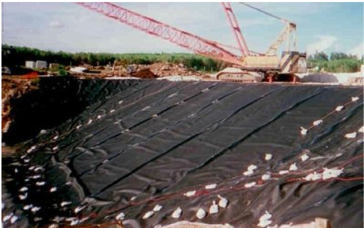
Landfill Cap – Remediation Project.
