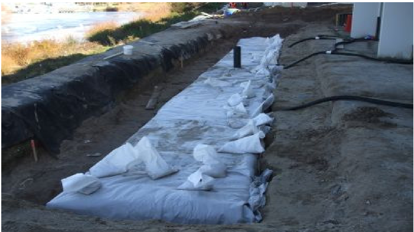
Completed system wrapped in Geotextile ready for backfilling.
